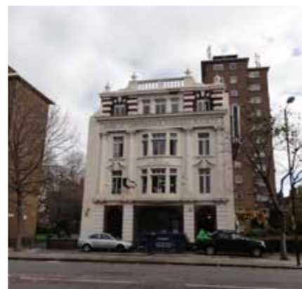
Sons of Temperance Building, Blackfriars Road
