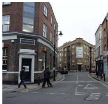
Former warehouse buildings on Morocco St
