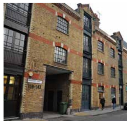
Formal warehouses on Tanner Street
