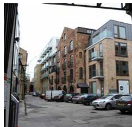
Views into internal block space
