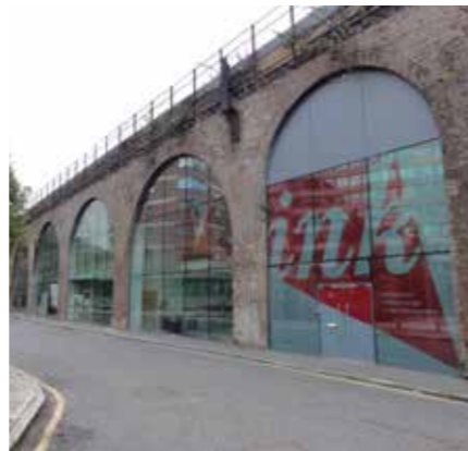
Development of railway arches for commercial use
